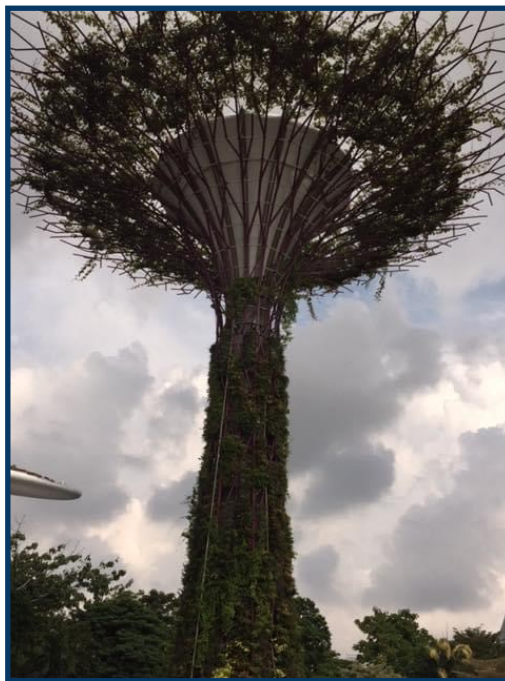
The Plants covered pillars in Garden at the Bay
